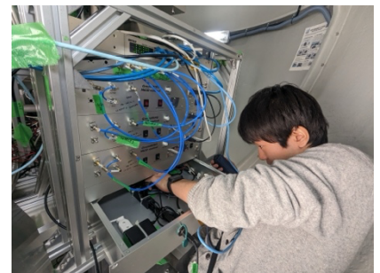
Fig. 1. Installation of new DAQ system.
